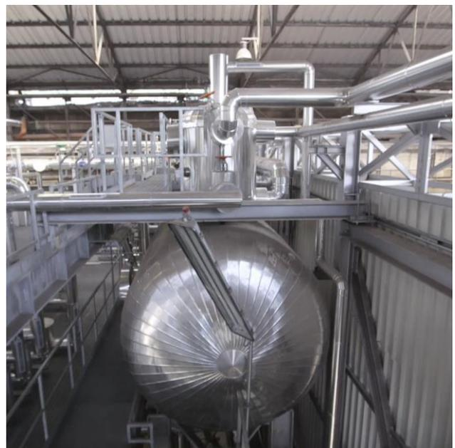
Steam accumulator and steam pipes. Source: ORI MARTIN
