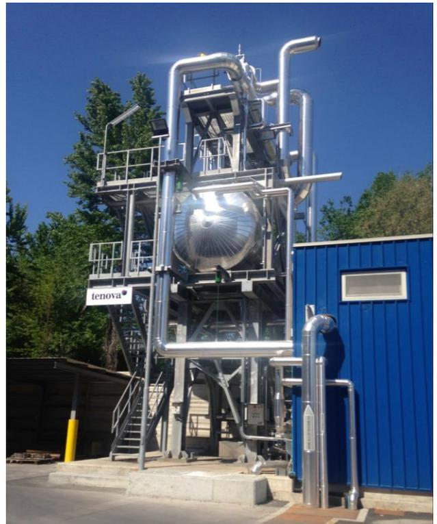
Heat substation for heat delivery to the district heating network operated by A2A. Source: ORI MARTIN
