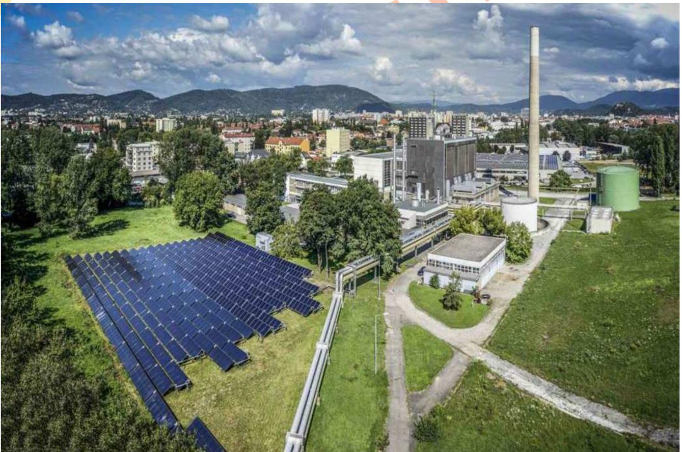
Test field of 2500 m<sup>2</sup> located in Graz for different solar collector's testing and selection of most suitable one for the large scale solar plant to be built in Kremsmünster. Source: Solid
