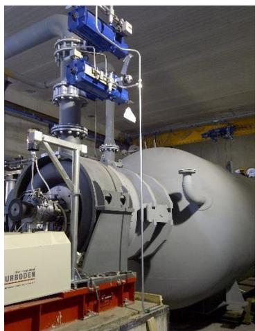
**Figure 5: Turbo-generator with Organic Rankine Cycle. Source: ORI MARTIN**
