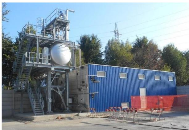
**Figure 4: Exchange unit with A2A heat district heating. Source: ORI MARTIN**
